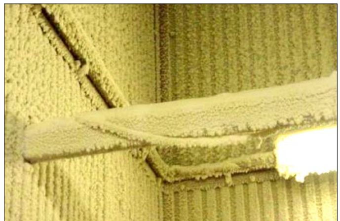
Figure 9. Sawdust clinging to horizontal and vertical surfaces
