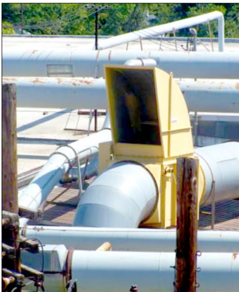
Figure 10. Abort gate in duct
