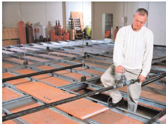
A technician adjusts a sprinkler that’s part of a 3M facility that tests its new clean agent: Novec 1230.
